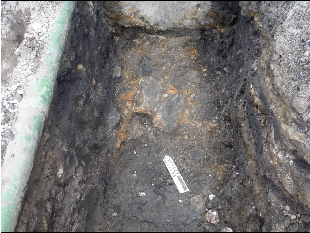
Figure 15. The rubble core of Hadrian's Wall. The large metal water pipe can be seen at the top of the photo. (Scale = 0.25m).
