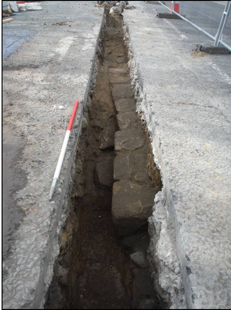
Figure 9. View looking north-west across Trench 1 with Hadrian's Wall (345) in the trench's south-west facing section. (Scale = 0.5m graduations).
