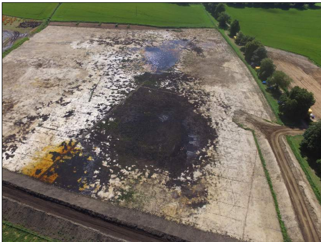
Figure 4. Aerial view of Wetland Basin 1, looking south.
